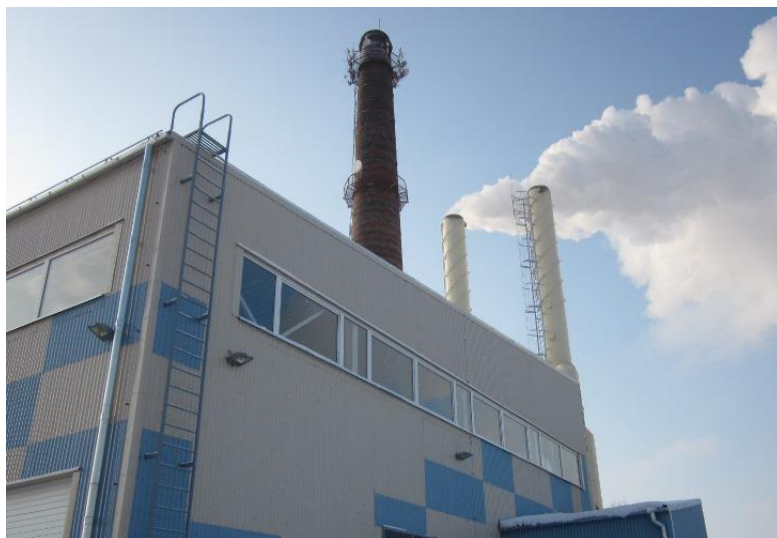
Biomass boiler-house in Tukums City
